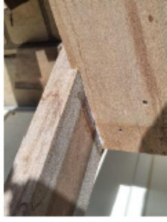
This is a key factor of the build, this image on the left is indicating and showing the rebated joint, as the seat component is slightly conjoint and merging with the right front leg with a "truss head" screw and more PVA wood glue keeping it in place.
